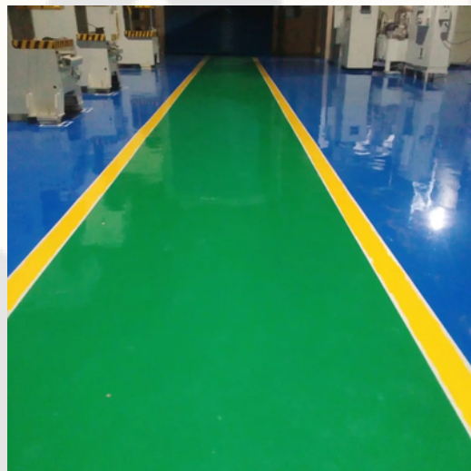
EPOXY FLOOR COATING
