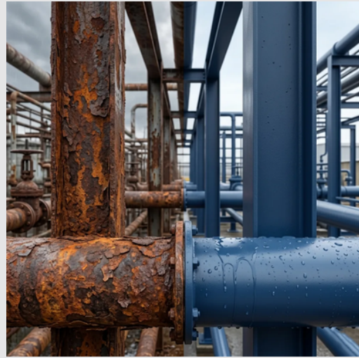
ANTI CORROSIVE PAINT COATING
