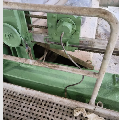
PU ANTI CORROSIVE COATING
