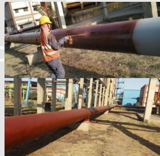
ANTI CORROSIVE EPOXY COATING FOR EXPOSED STEEL
